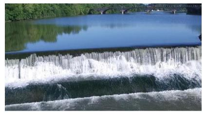
April is Low Head Dams Public Safety Awareness Month! According to the American Society of Civil Engineers (ASCE), "A low head dam is a manufactured structure, built in a river or stream channel, extending fully across the banks. A low head dam is designed and built such that water flows continuously over the crest from bank to bank. If water levels rise downstream,
